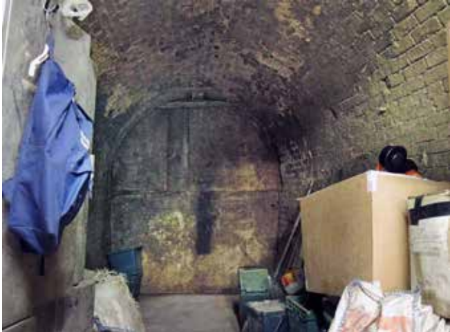
The surviving part of the tunnel now used for storage. Photo courtesy of Dr Ian Dungavell/Friends of Highgate Cemetery Trust
